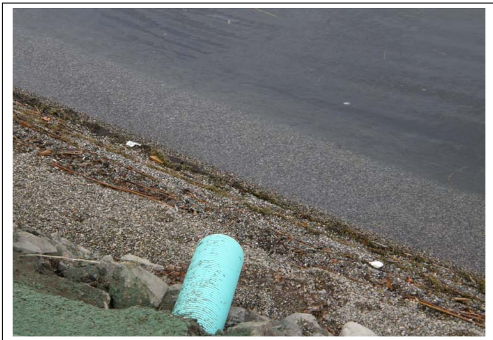
Photo 2: The portion of the Granular Beach habitat requirement adjacent to the linear planting bench was completed in the fall of 2007. It will be extended along the remainder of the linear planting bench to be constructed in 2008 (photo Dec. 5, '07).
