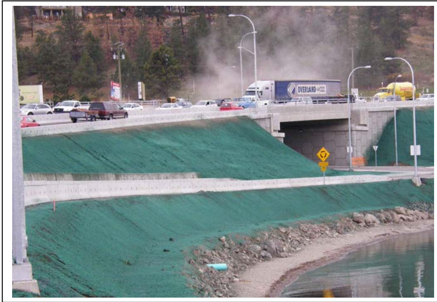
Photo 1: The south-westerly portion of the linear planting bench along the Campbell Road Interchange was constructed and hydro-seeded in the fall of 2007. It will be planted to native willows in the spring of 2008 (photo Nov. 14 '07).
